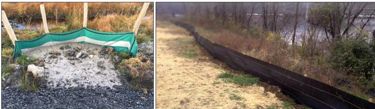
Figure 1-2 Silt fencing measures (Source: SSI Environmental (left) and Thrace Group (right))
