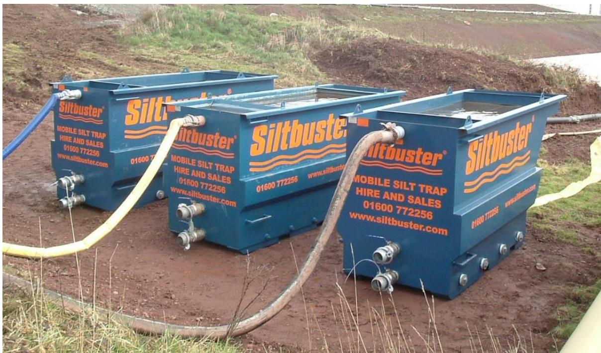
Figure 1-3 Temporary site settlement tanks (Source: Siltbuster)
